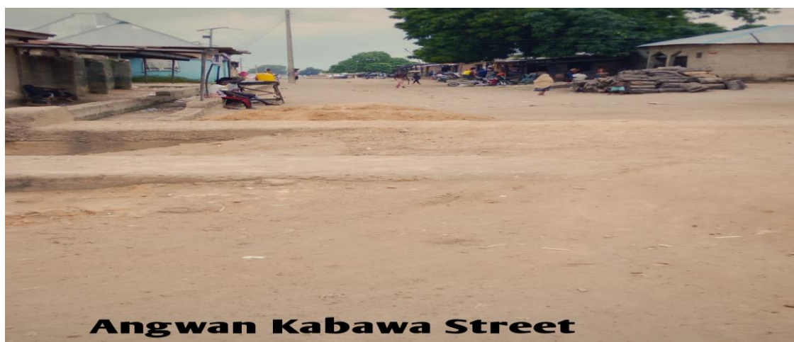
Figure 3: Angwa Kabawa Street - Constituency road project
